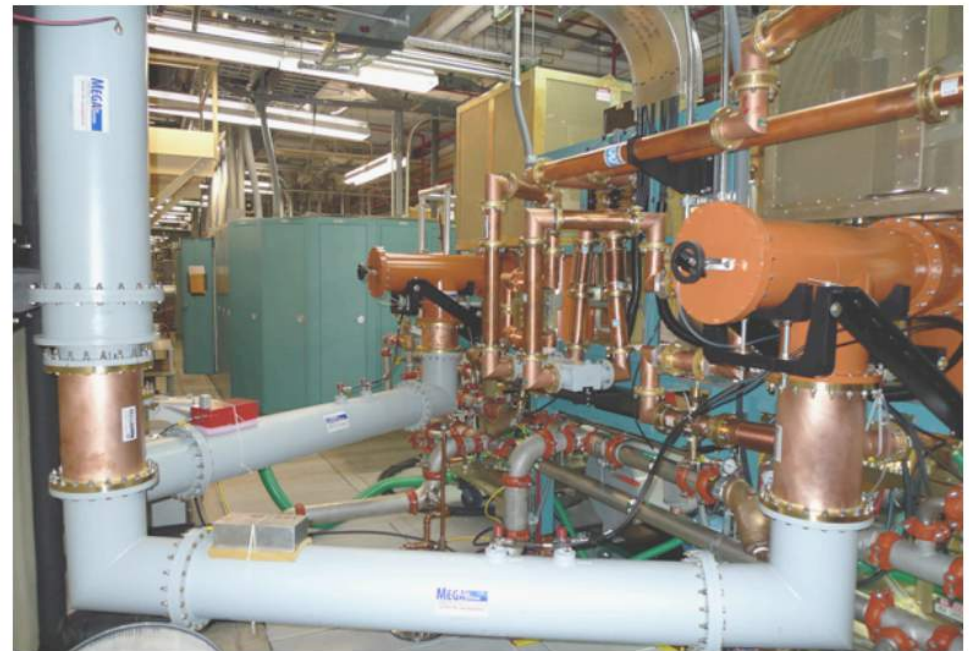
Figure 2: Coaxial feeders from PAs to branch hybrid
