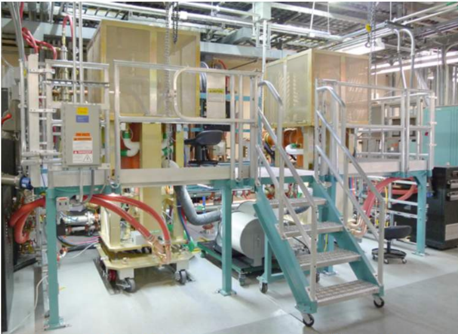
Figure 3: Dual FPAs with Diacrodes ® installed
